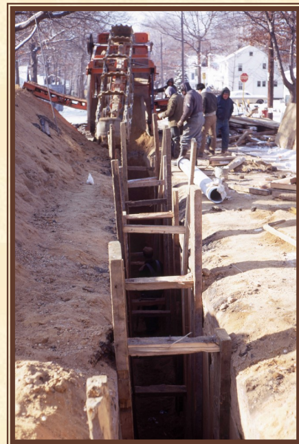
Construction of Sewer Lines
